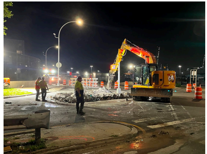
Demolition of median island at Columbia Street
