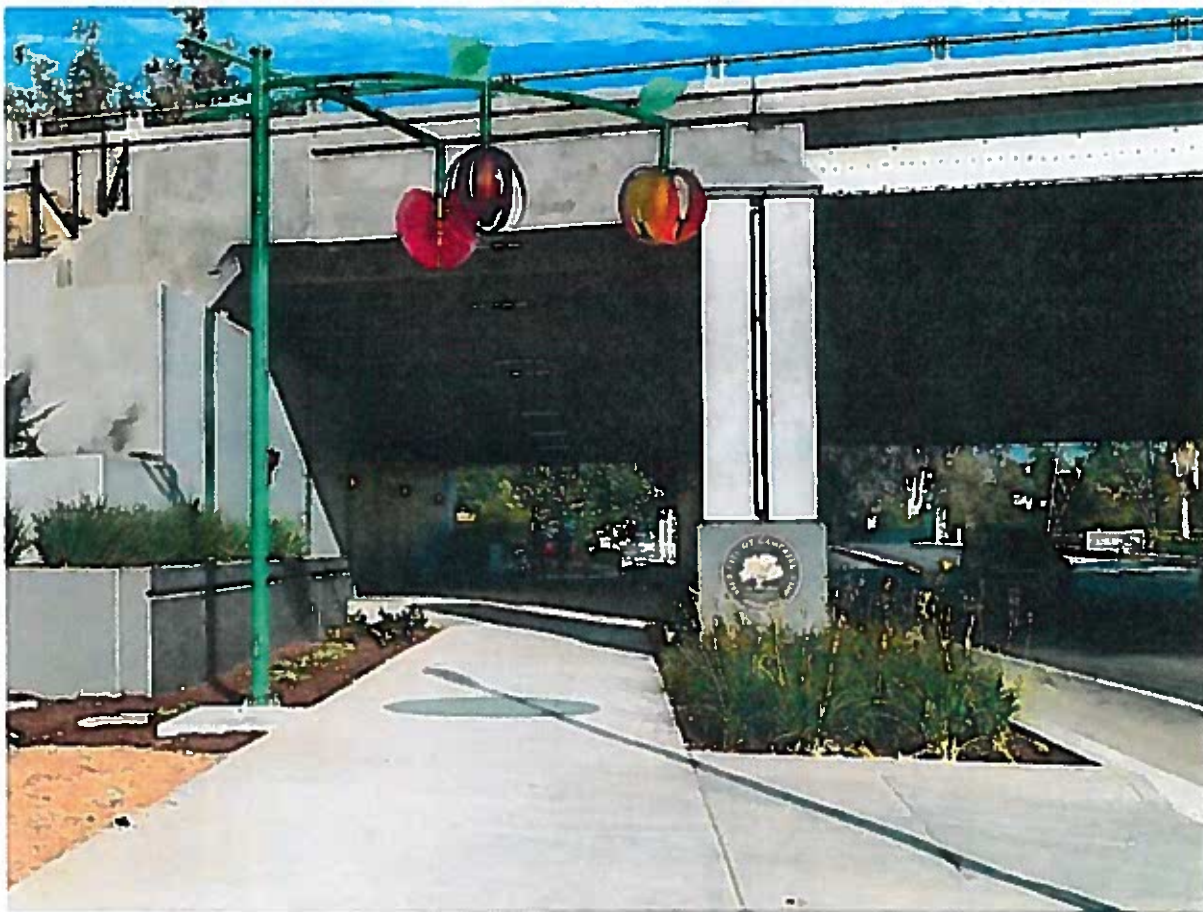
The portals create a pleasant entryway to downtown Campbell. | City of Campbell
