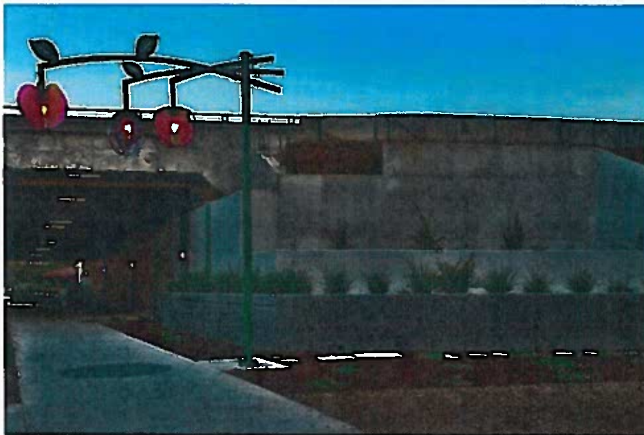
The East Campbell Avenue Portals opened this week | City of Campbell
